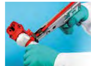
Tighten cable ties
