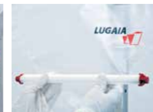
Press round stick into Omega Profile
